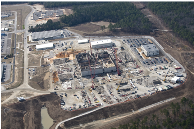
MOX Fuel Fabrication Facility
