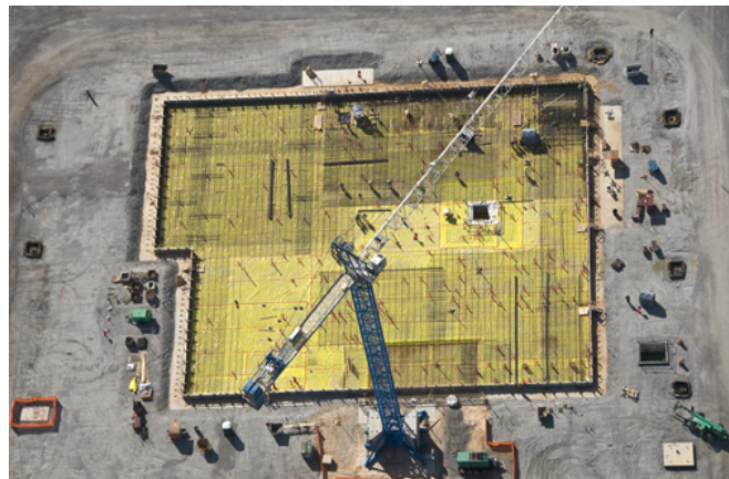
Waste Solidification Building
